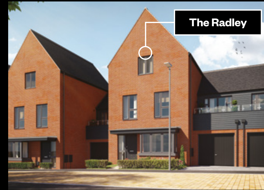
The Radley 4 bedroom semi-detached and mid-terrace home with study and drive-through carport
