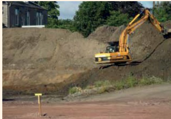
The process required ground testing at every 300mm infill layer before the subsequent layer was placed, ensuring solid compaction to support the new building foundations.
